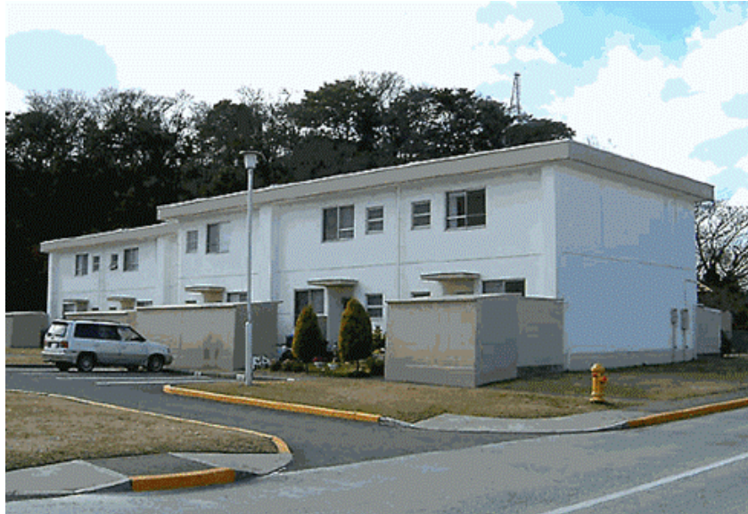
Figure 17. Example of a two-story townhouse at Yokosuka Naval Base
